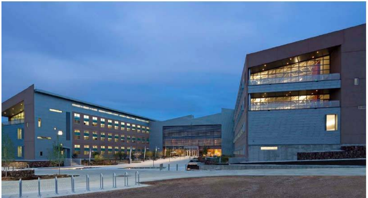
“Research Support Facility (RSF) , NREL” - USA
