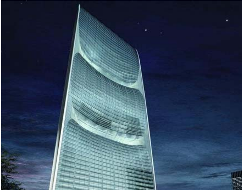
“Pearl River Tower” – Guangzhou, China
