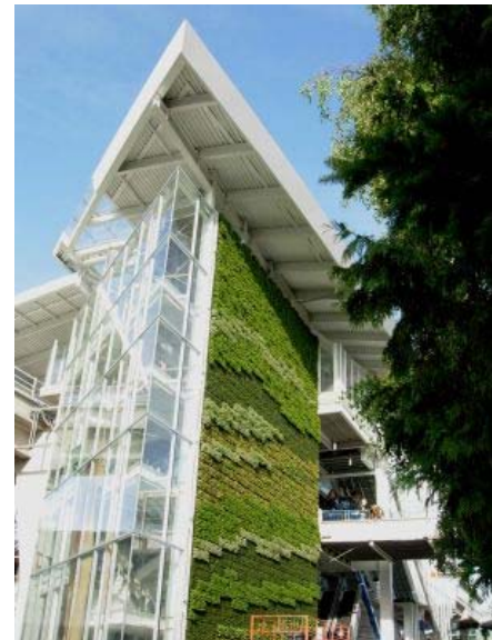
Figure C1-7-1.4 : Example of exterior green wall (Sexton,2013)
